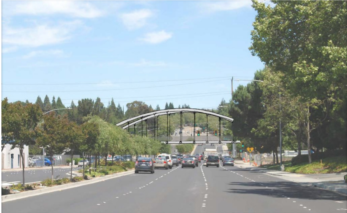
Crow Canyon Road – Tied-Arch-Stayed – looking east
